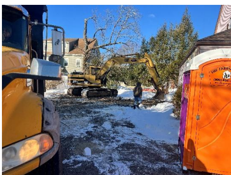
Ground was broken for the new addition on February 12, 2026.
